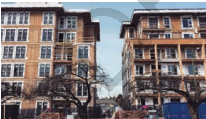
Multi-family timber frame construction, Cambie Street (Source: Aaron Lao)
